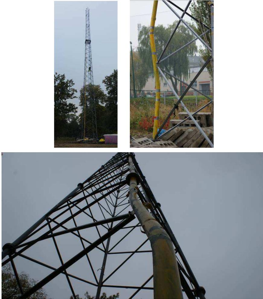
FIG. 1. The general view of the tower (top left), failure mode of the leg in the lowest section (top right and bottom).
